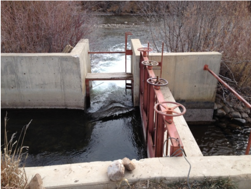
Photo 2: Gunnison River/Ohio Ditch headgate.
