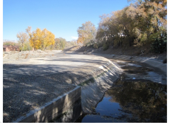
Grand Valley Irrigation Company lined canals
