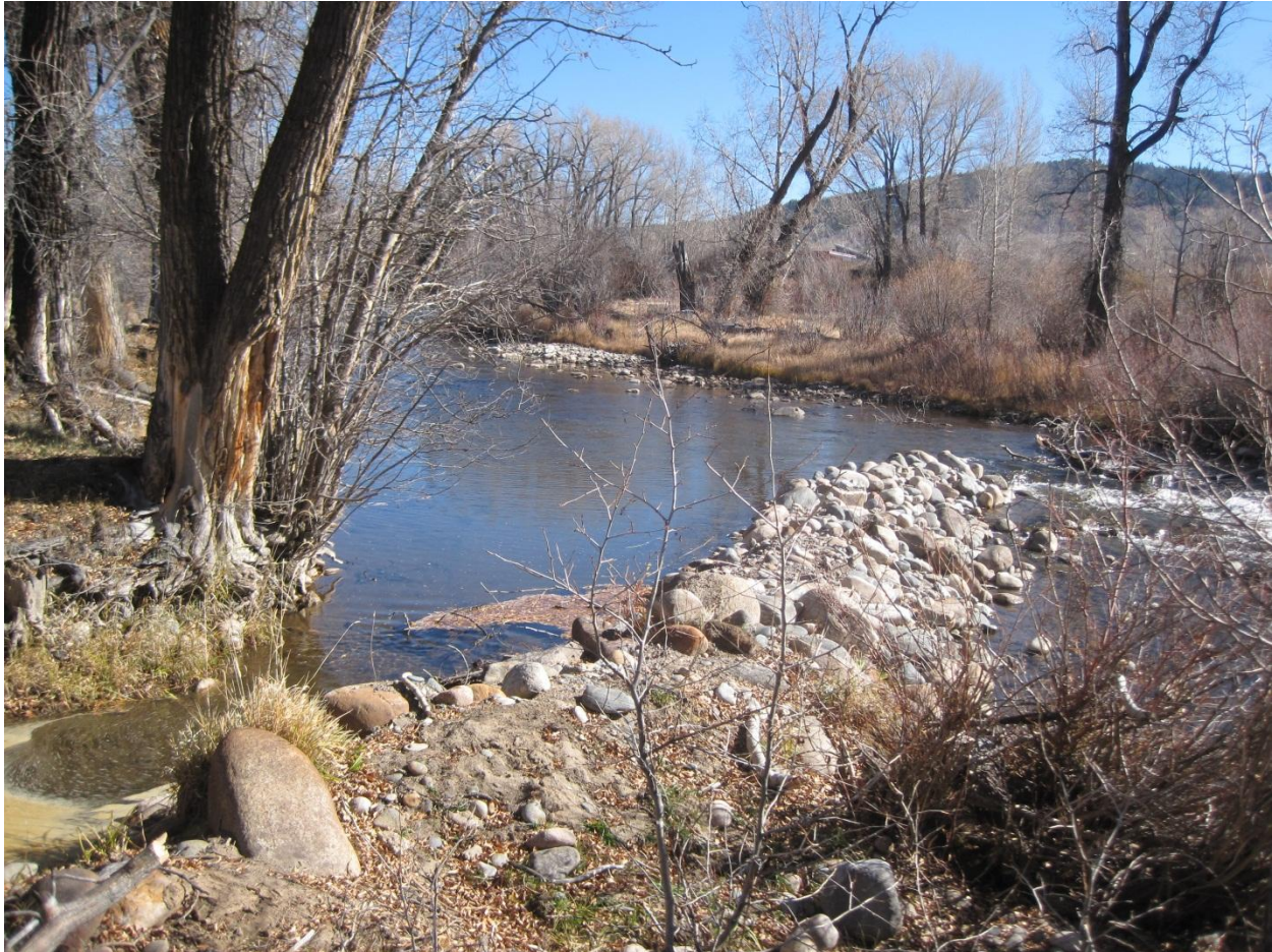
Photo 2: Ekhart Ditch diversion structure on the Elk River.
